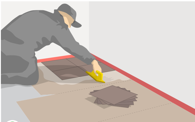
3 Final floor application (glued)
