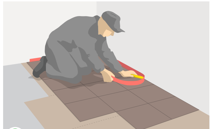
4 Perimeter insulation barrier cut
